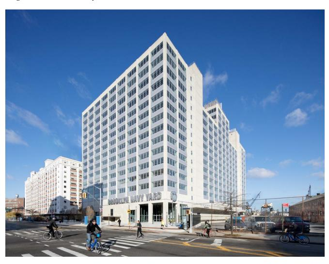
The building was rapidly constructed in 1942 as a 16-story reinforced concrete structure. The windowless lower 11 floors provided warehouse storage, while the upper floors served as offices for the Yard's Commandant and the US Navy's oversight of the North Atlantic Fleet during WWII. The building is a part of the National Register Brooklyn Navy Yard Historic District.
